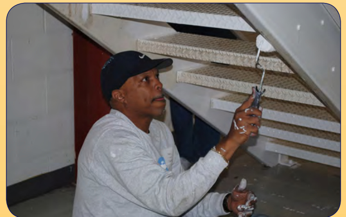
CSX volunteer painting stairs
